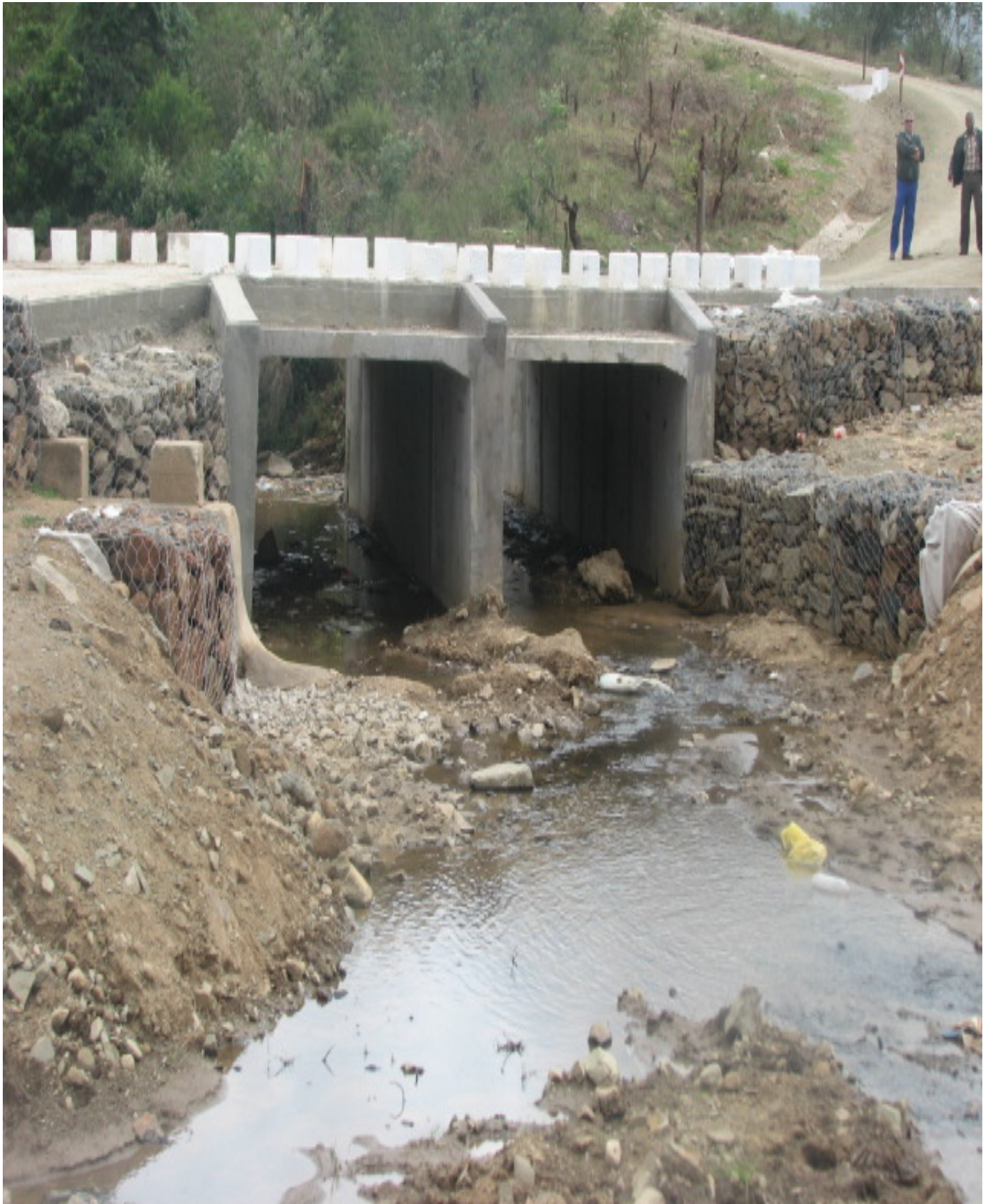
NEW NDLOVINI LOW-LEVEL BRIDGE – VALUE – R800 000.00
